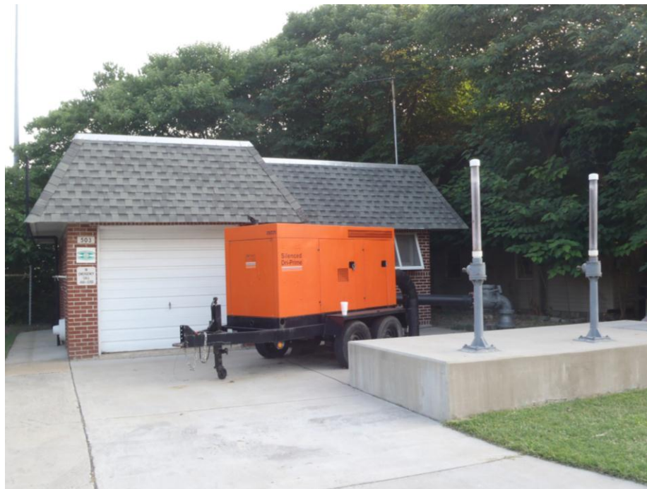
Figure 119-2. Park Ave Pump Station
