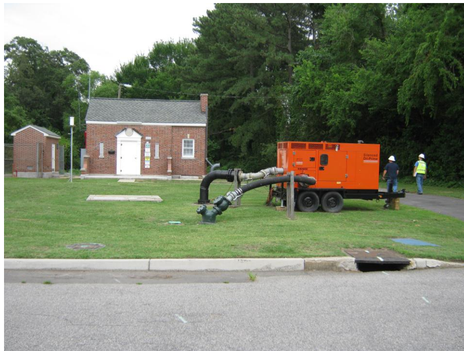
Figure 113-2. Luxembourg Ave Pump Station
