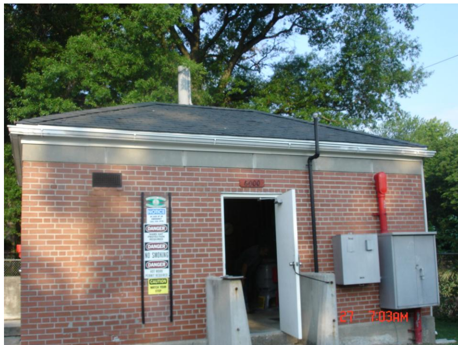
Figure 219-2. Newmarket Creek Pump Station
