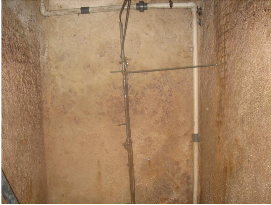
Figure 145-3. Rodman Ave Wet Well Walls
