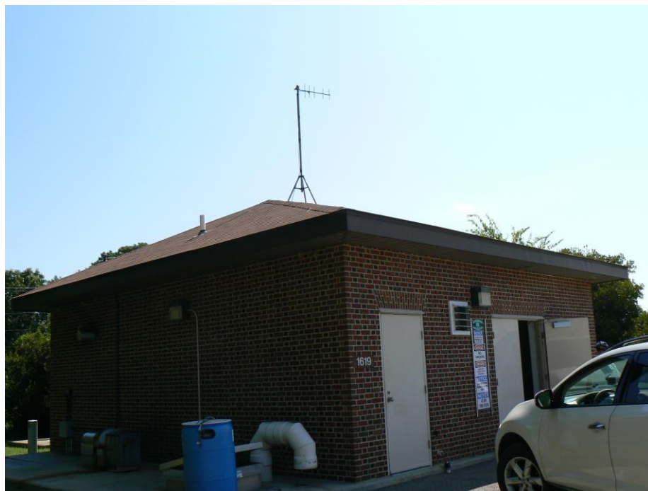
Figure 227-2. Fort Eustis Pump Station
