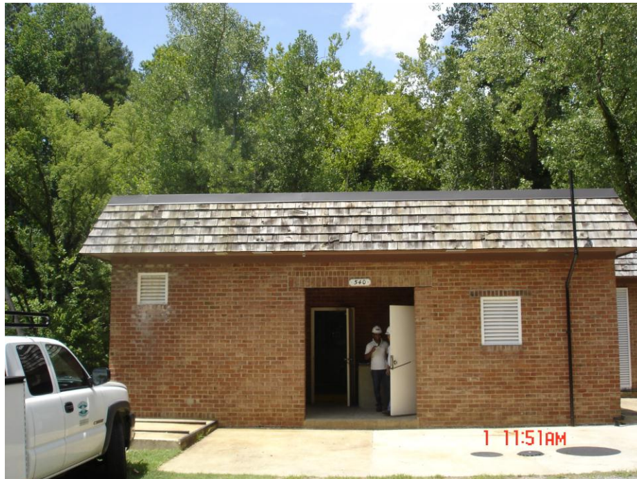
Figure 226-2. Williamsburg Pump Station
