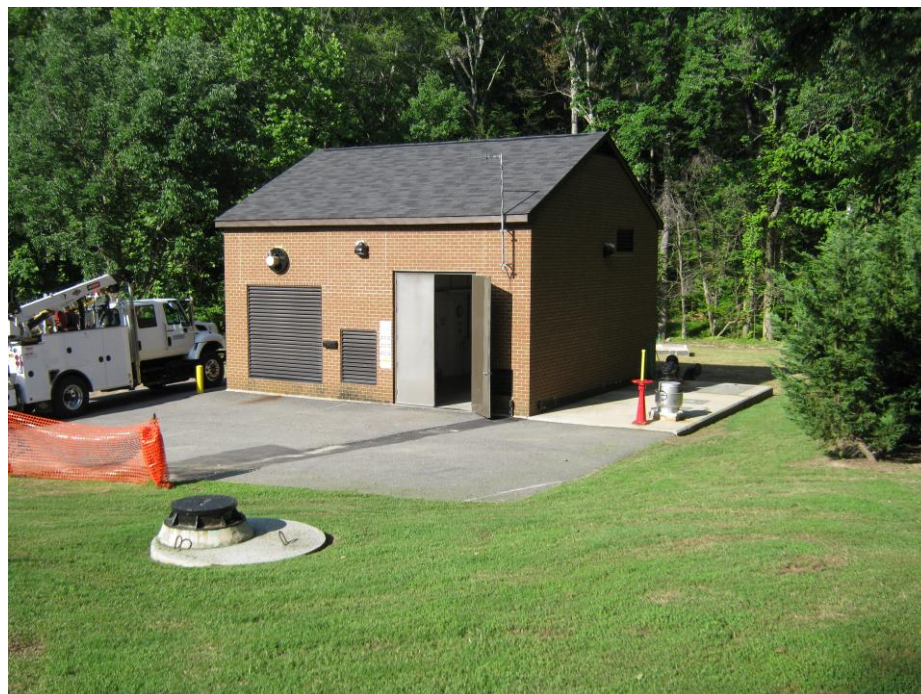
Figure 233-2. Lodge Rd Pump Station
