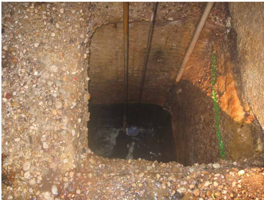
Figure 145-4. Rodman Ave Wet Well Deck
