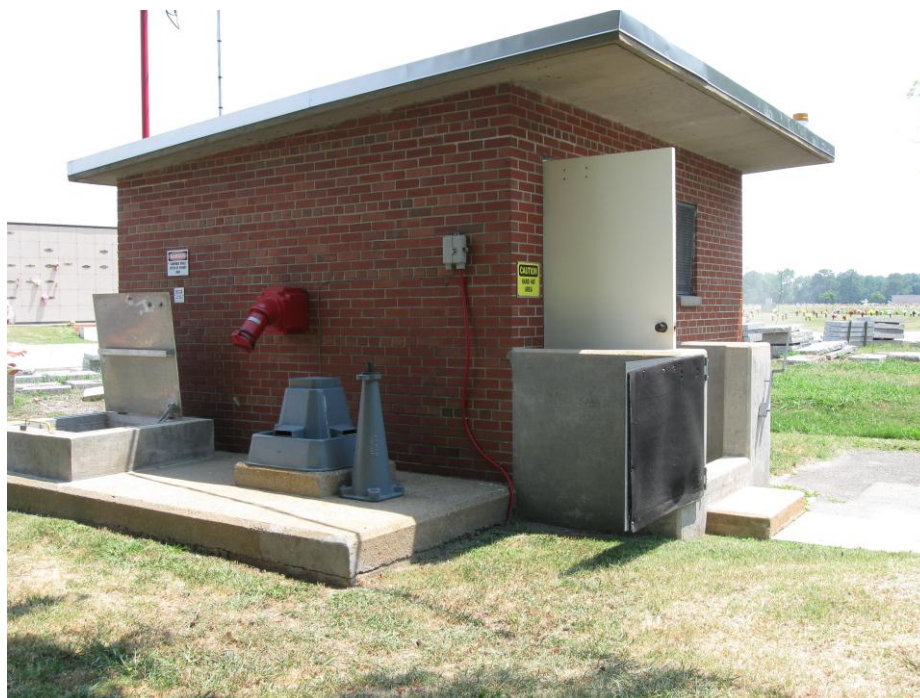
Figure 109-2. Dozier's Corner Pump Station
