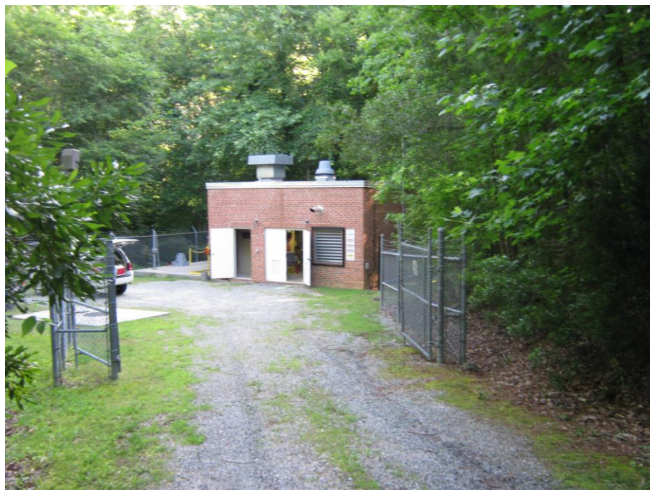
Figure 230-2. Rolling Hills Pump Station
