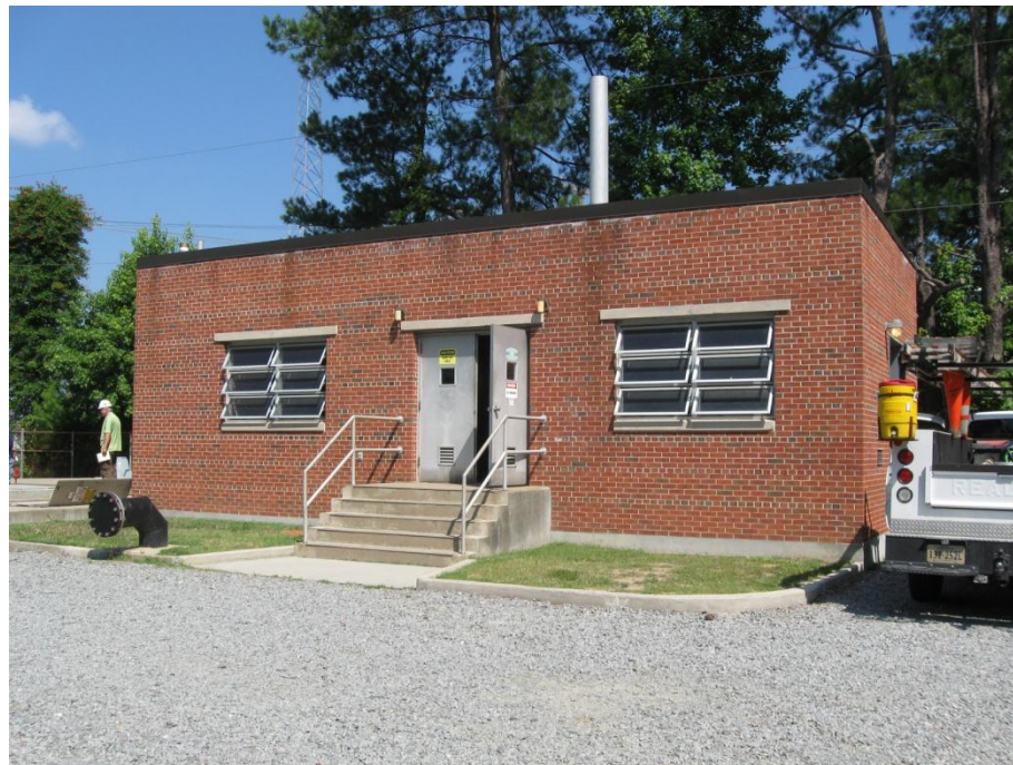
Figure 104-2. Cedar Lane Pump Station
