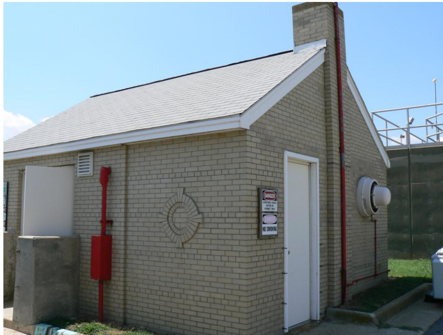
Figure 213-2. Jefferson Ave Pump Station
