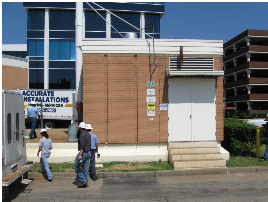
Figure 107-2. Colley Ave Pump Station
