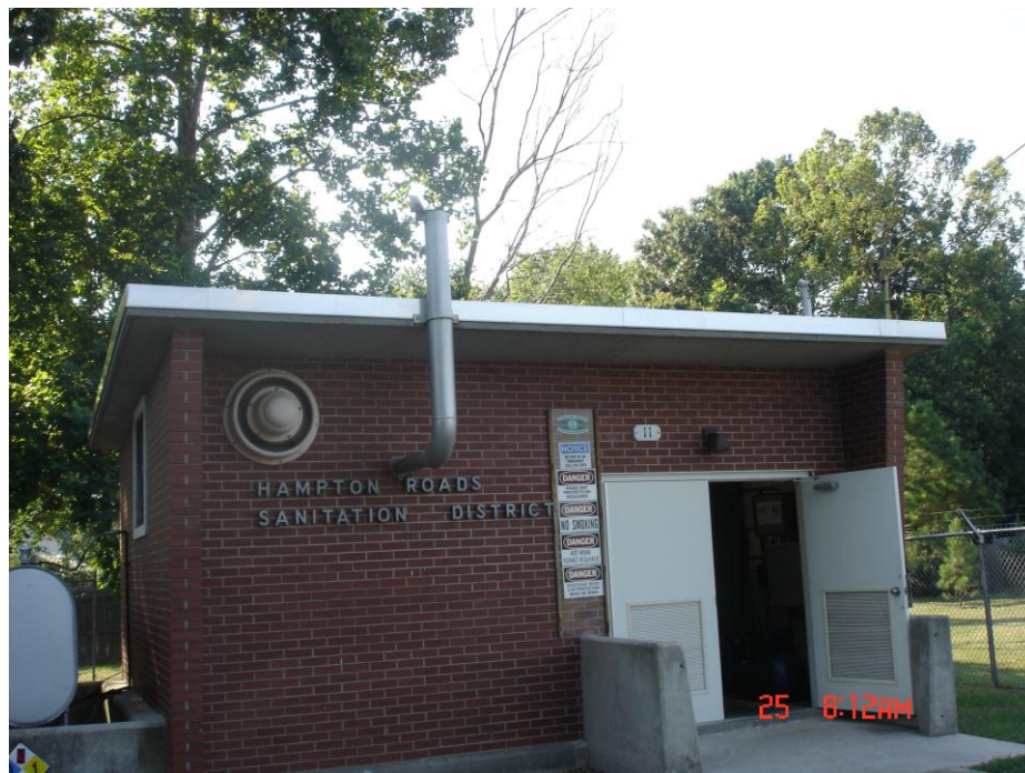
Figure 224-2. Woodland Rd Pump Station
