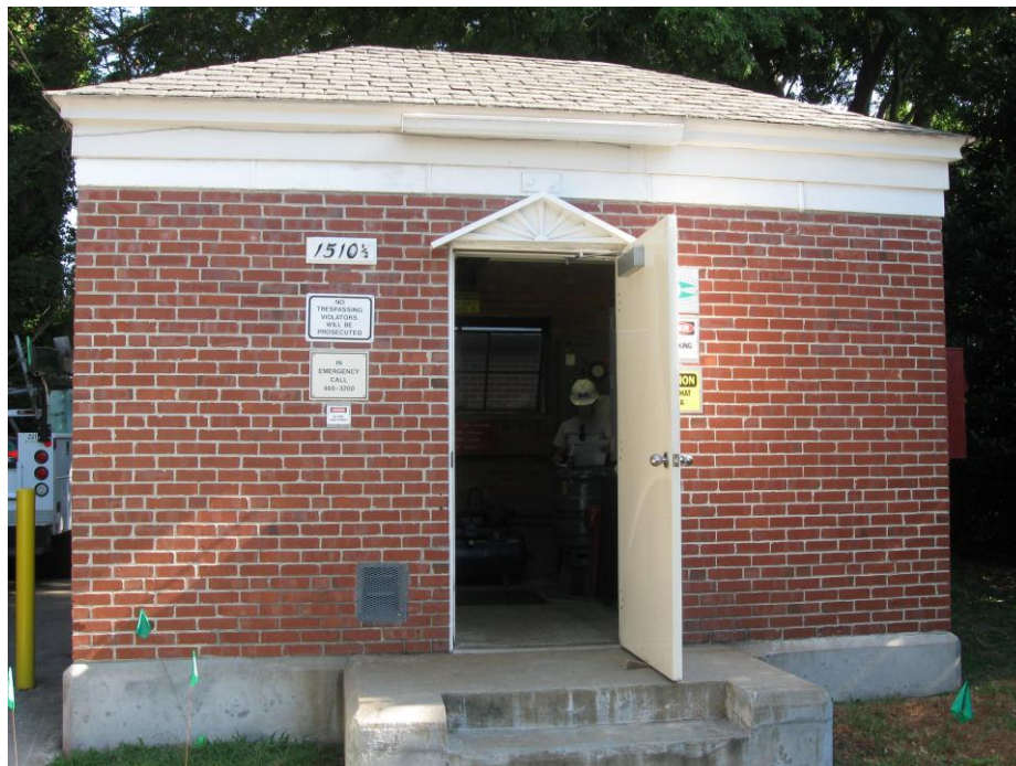
Figure 117-2. North Shore Rd Pump Station
