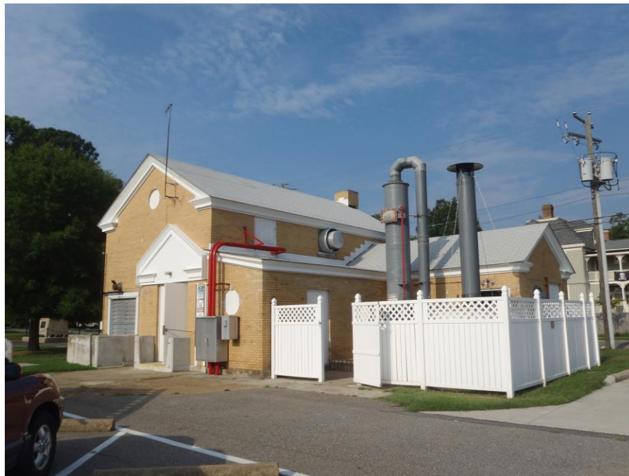
Figure 206-2. Bridge Street Pump Station
