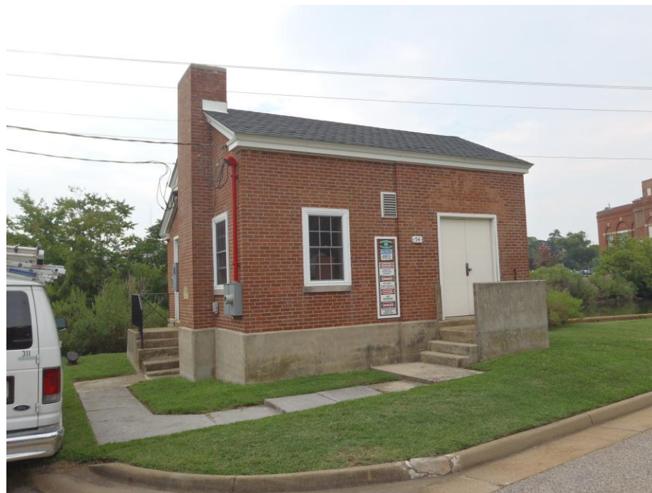
Figure 211-2. Hampton Institute Pump Station
