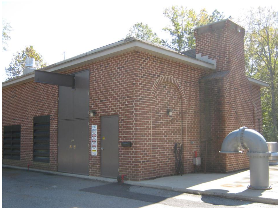
Figure 232-2. Greensprings Pump Station
