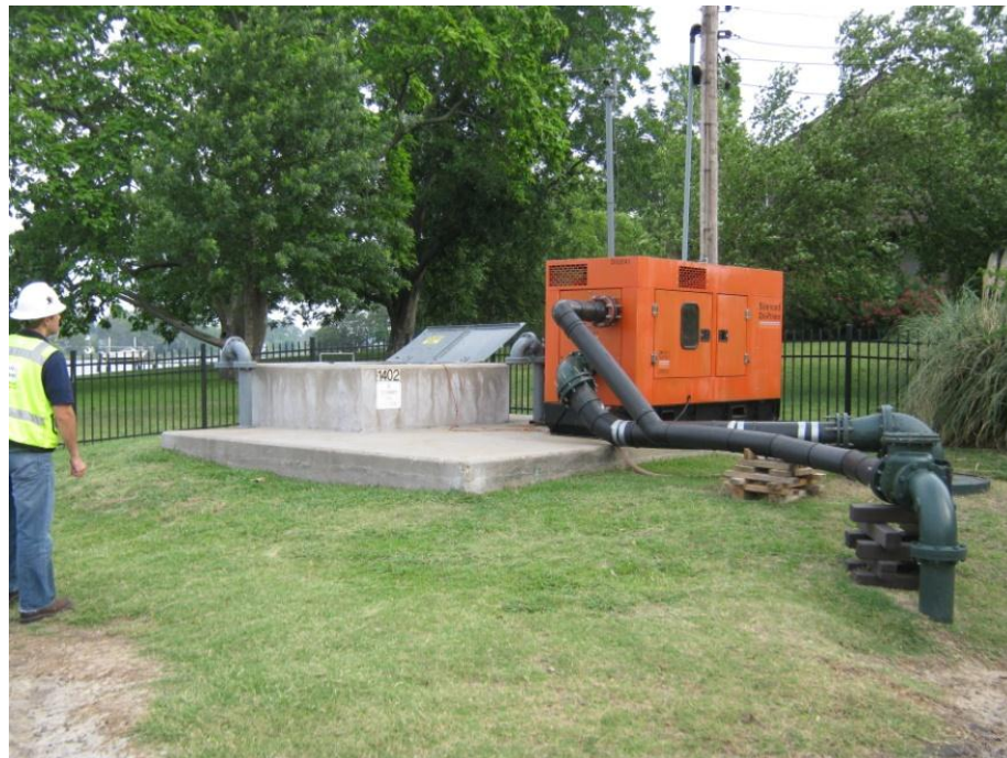
Figure 102-2. Ashland Circle Pump Station
