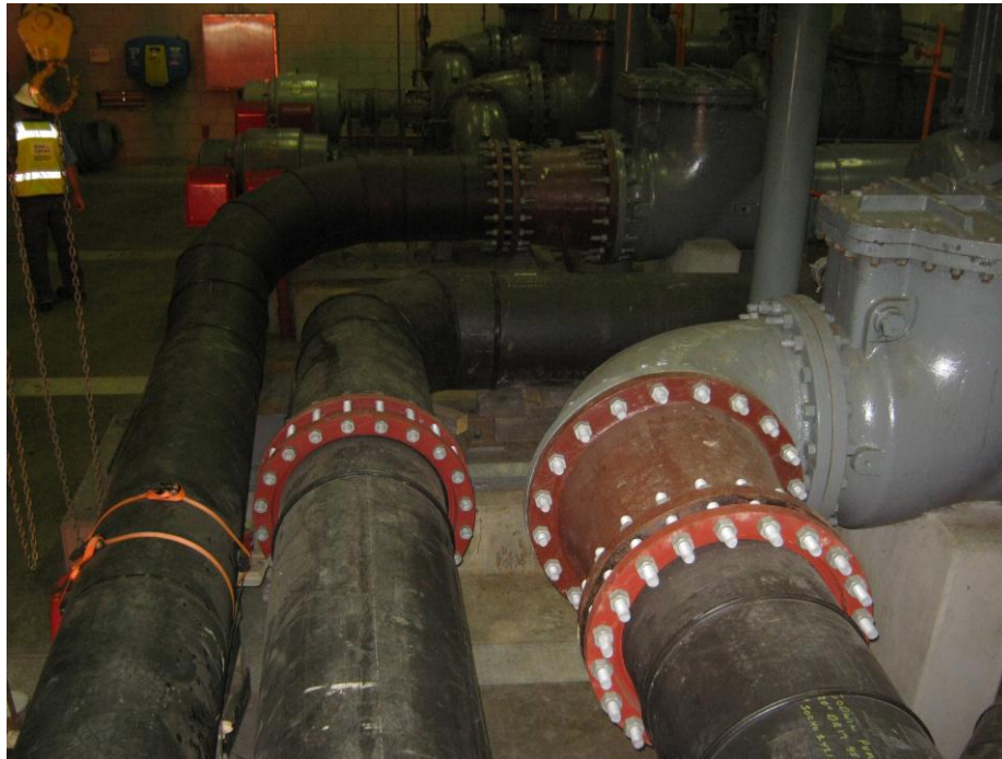
Figure 143-3. Shipp's Corner HDPE Diesel-Driven Pump Piping
