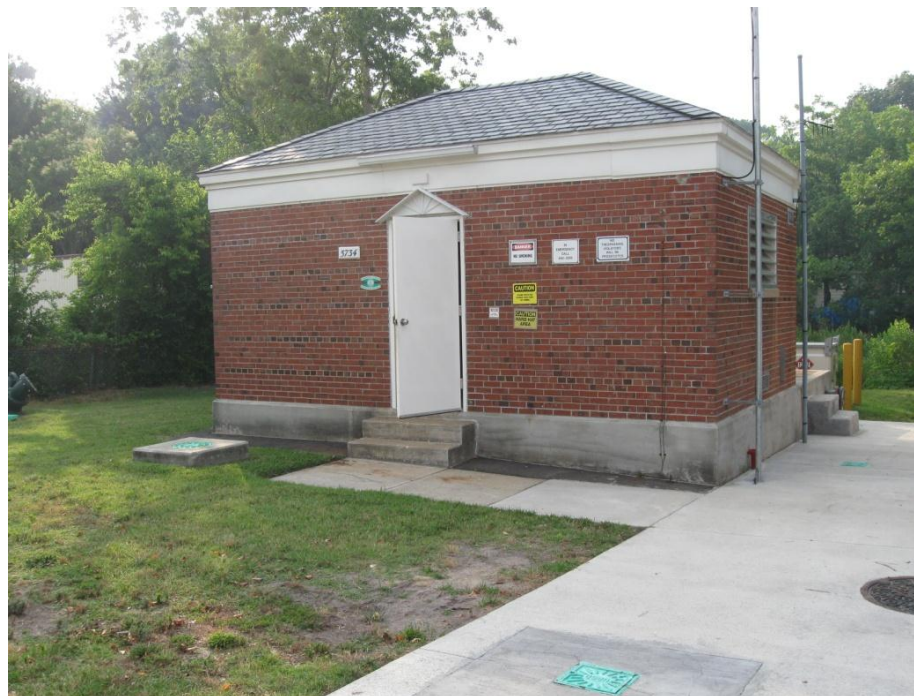
Figure 105-2. Chesapeake Blvd Pump Station
