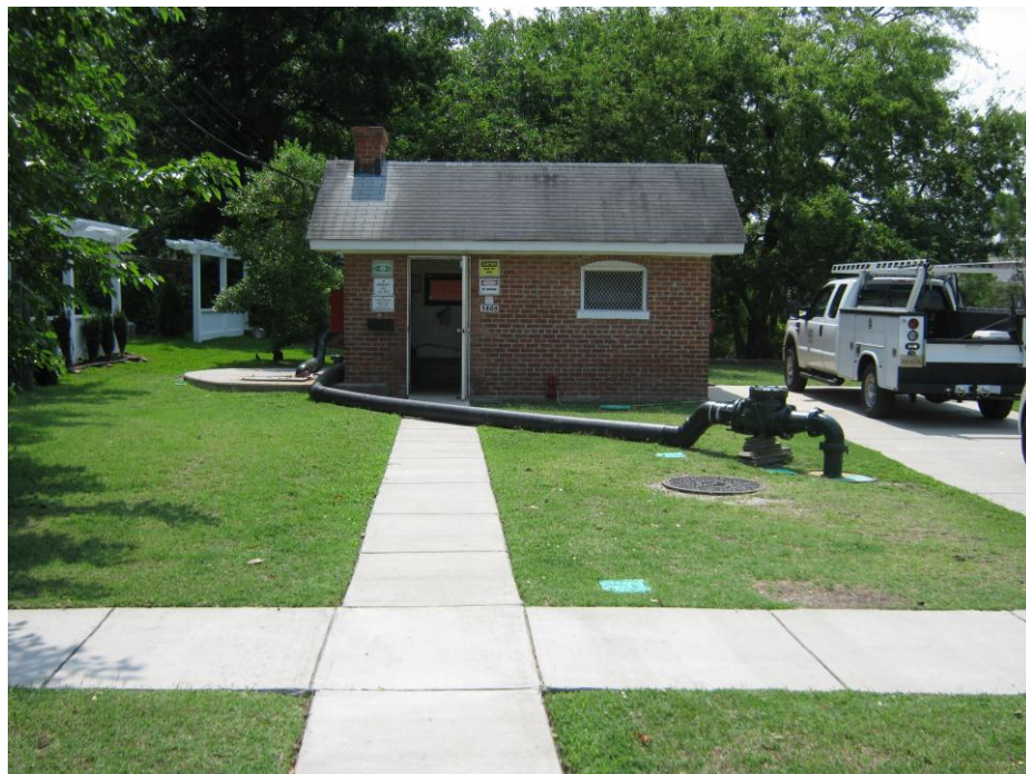
Figure 114-2. Monroe Place Pump Station
