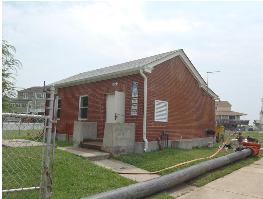
Figure 203-2. Bay Shore Lane Pump Station
