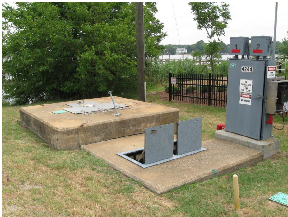
Figure 111-2. Granby Street Pump Station
