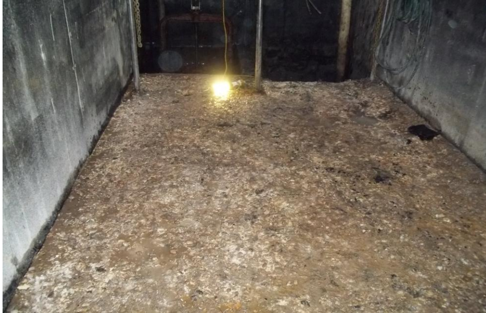
Figure 108-3. Dovercourt Wet Well Intermediate Slab
