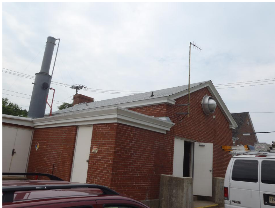
Figure 225-2. Willard Ave Pump Station
