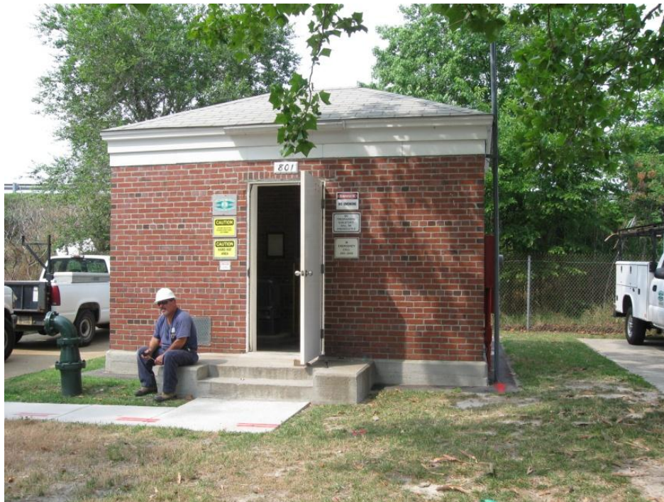
Figure 103-2. Bainbridge Blvd Pump Station
