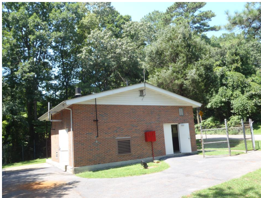
Figure 220-2. Normandy Lane Pump Station
