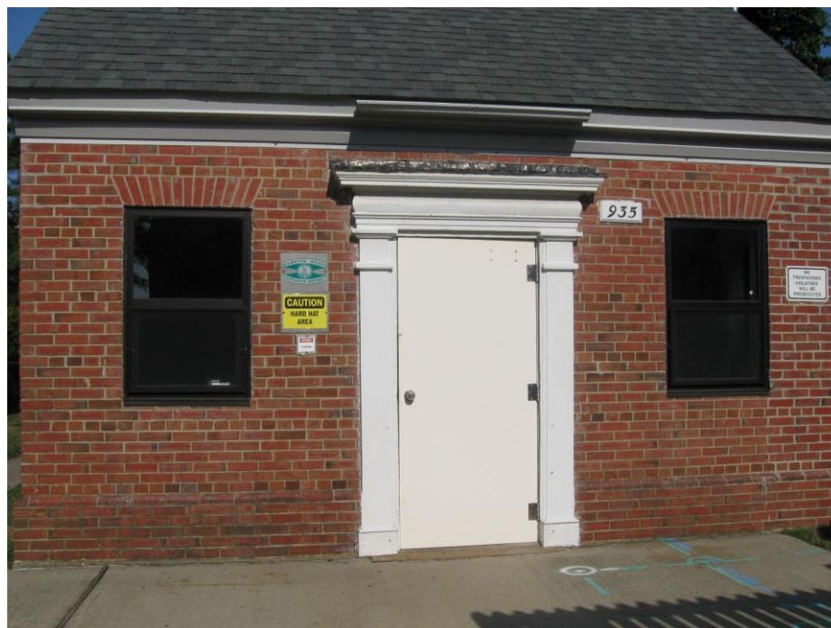
Figure 116-2. Norchester St Pump Station
