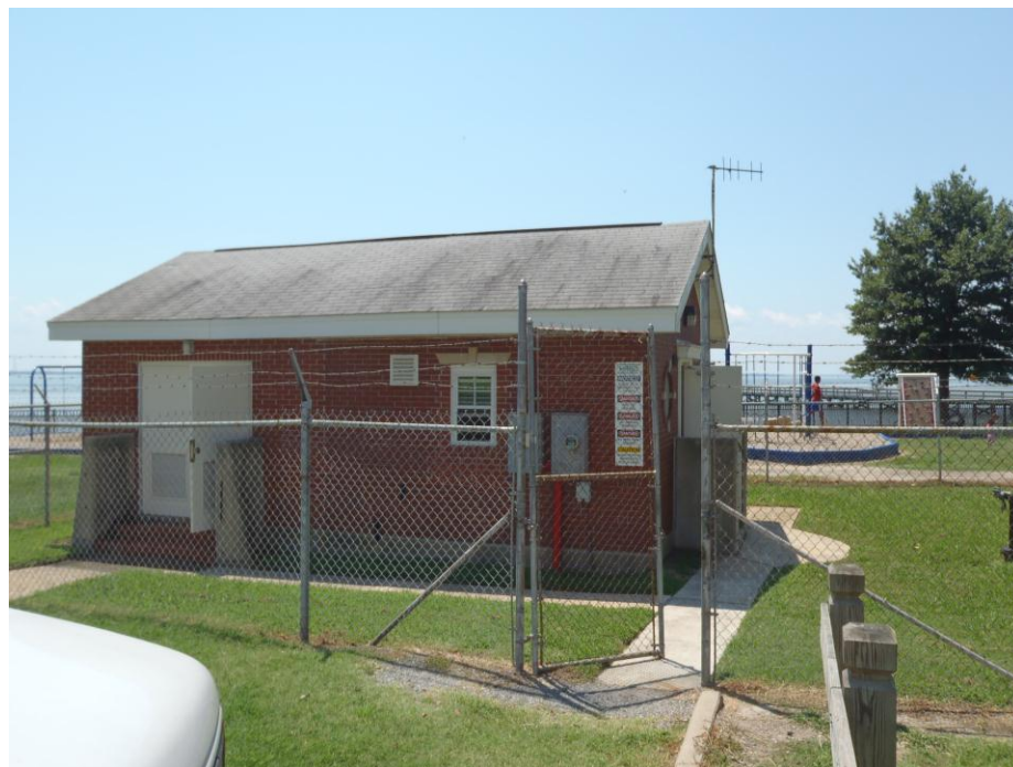
Figure 212-2. Hilton School Pump Station
