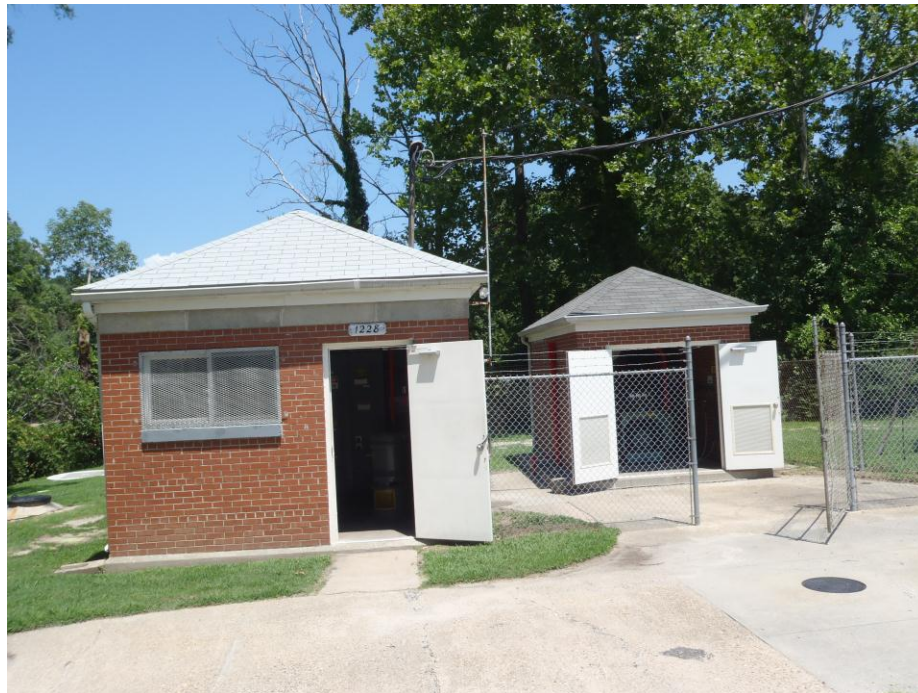
Figure 218-2. Morrison Ave Pump Station
