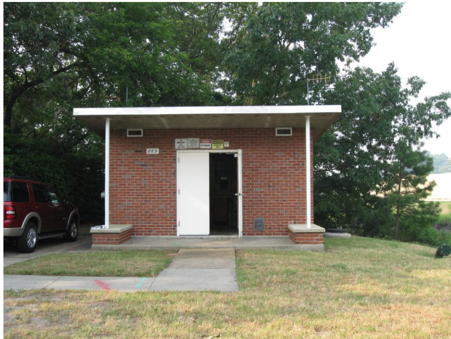
Figure 118-2. Norview Ave Pump Station
