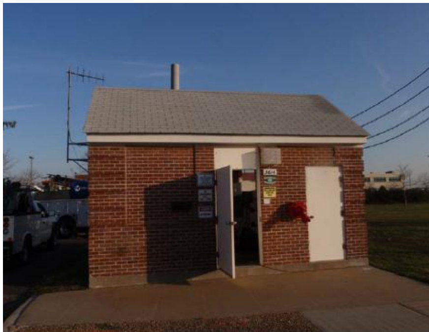
Figure 130-2. Virginia Beach Blvd PS
