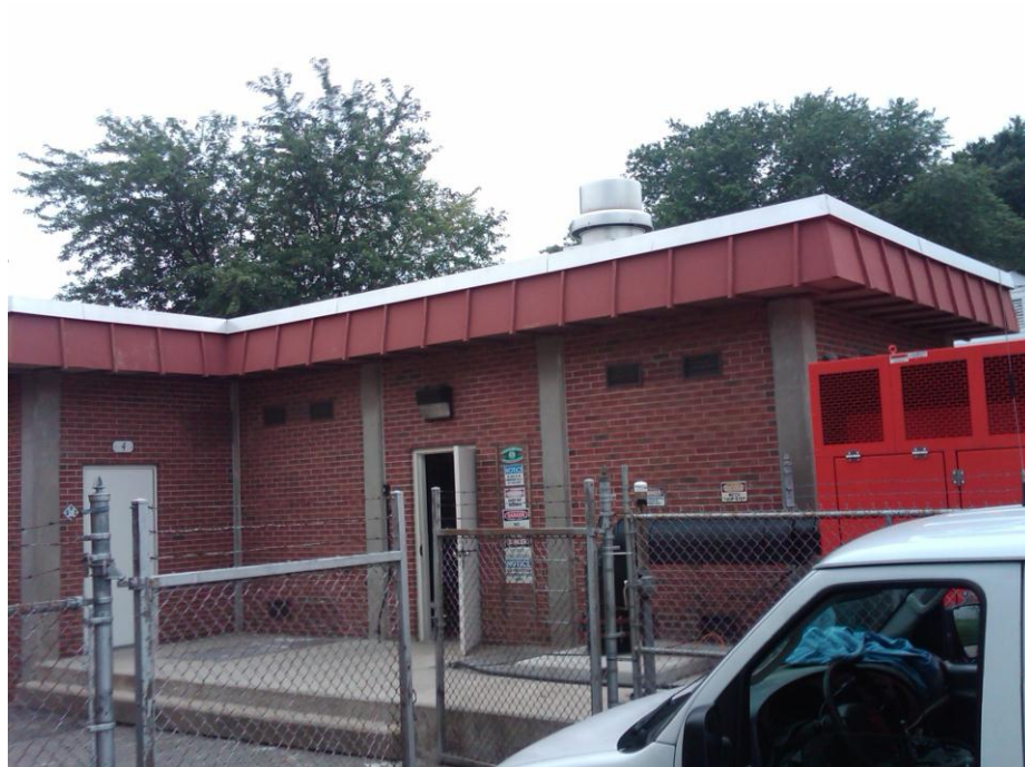
Figure 217-2. Langley Circle Pump Station
