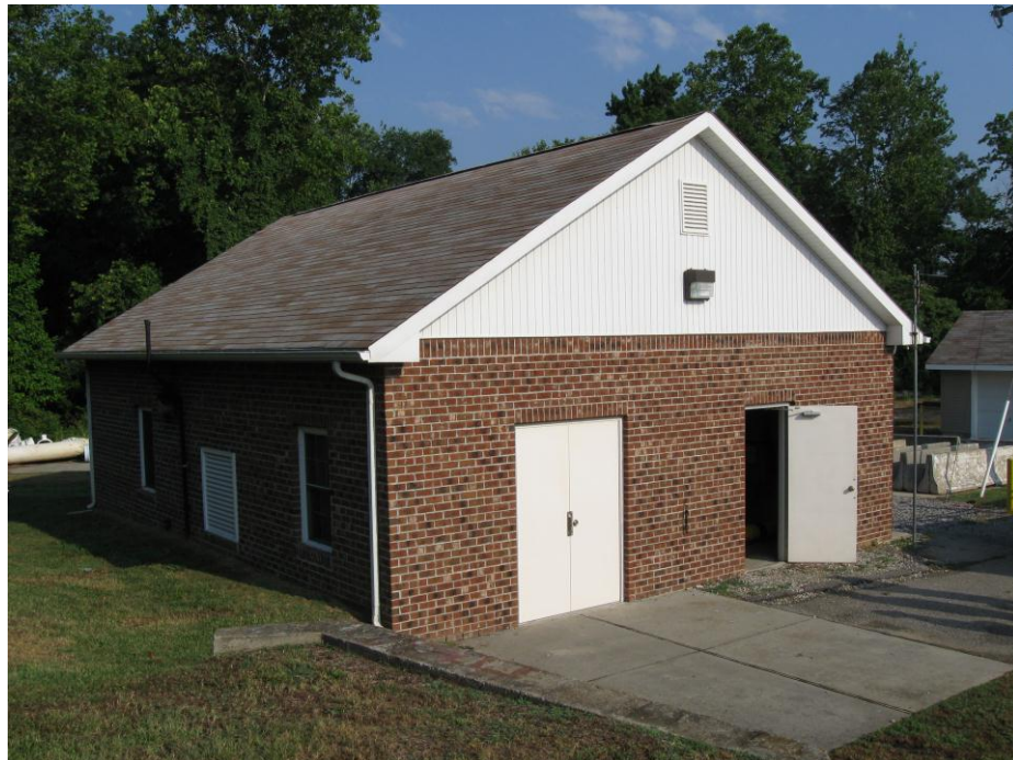
Figure 221-2. Patrick Henry Pump Station
