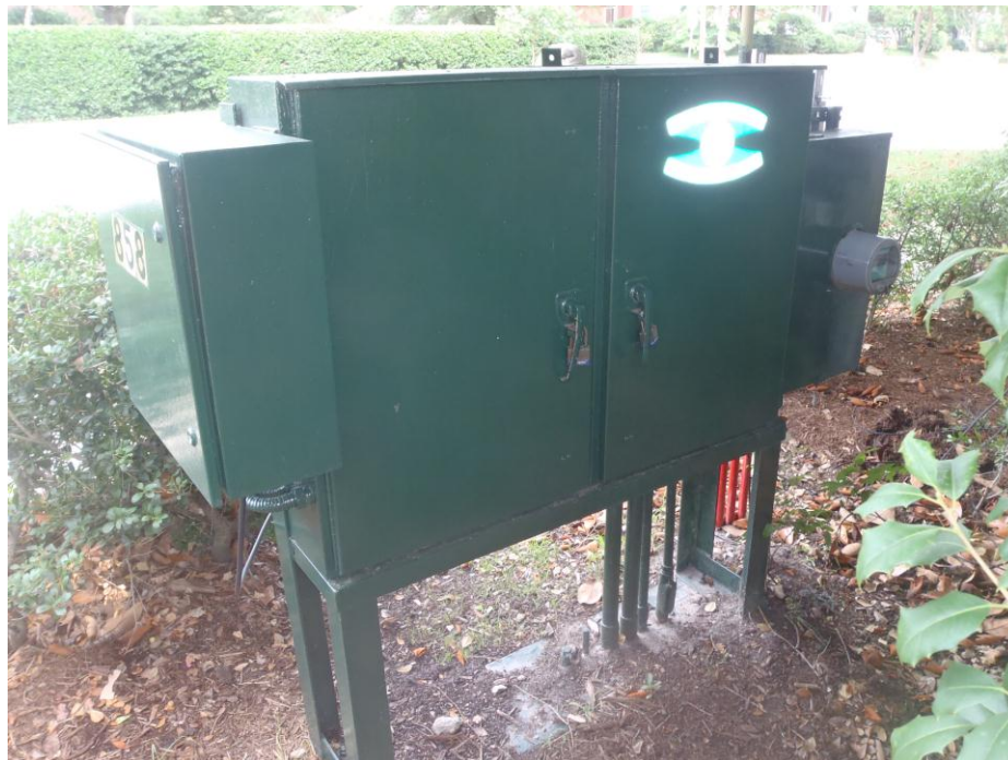
Figure 142-2. Jamestown Crescent PS
