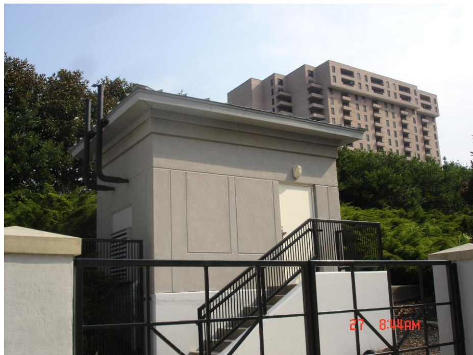
Figure 201-2. 25 th Street Pump Station
