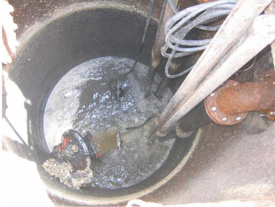
Figure 147-3. Chesterfield Blvd Wet Well
