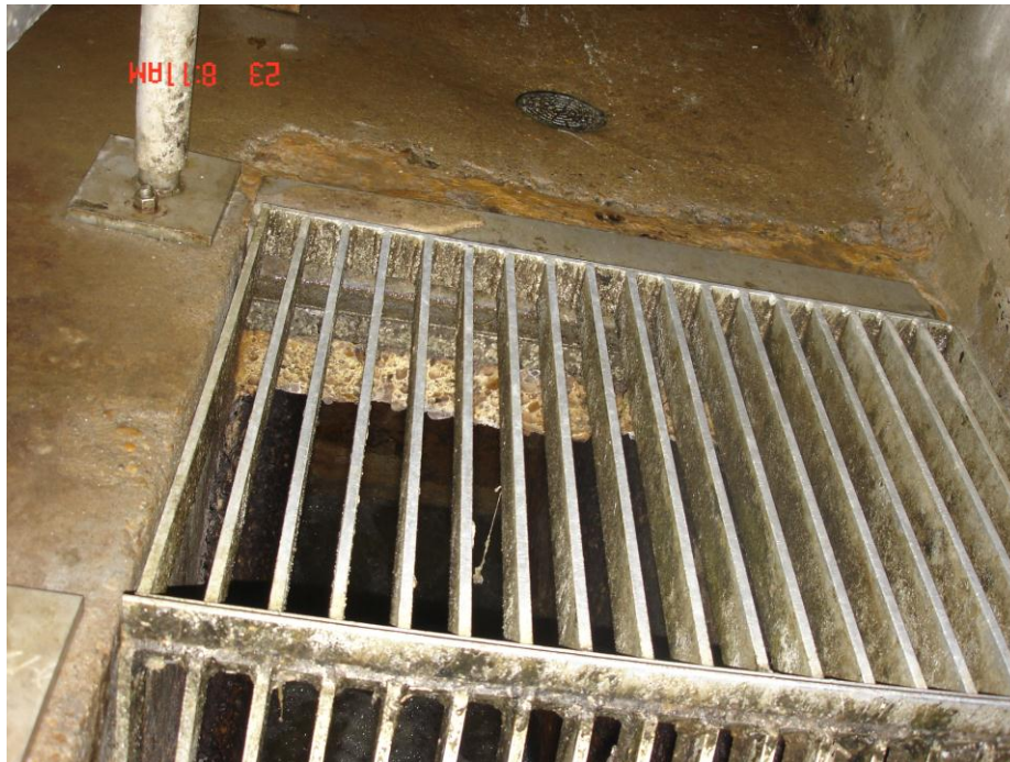
Figure 231-3. Fords Colony Wet Well Slab
