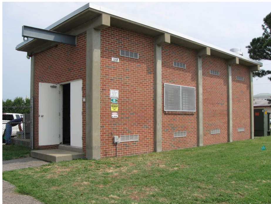
Figure 115-2. Newtown Road Pump Station
