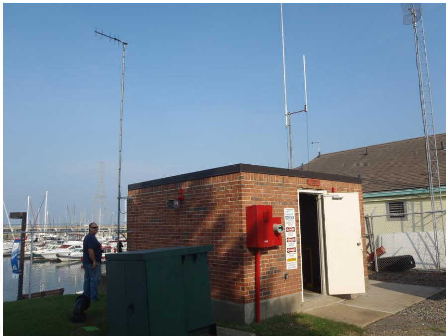
Figure 210-2. Ferguson Park Pump Station
