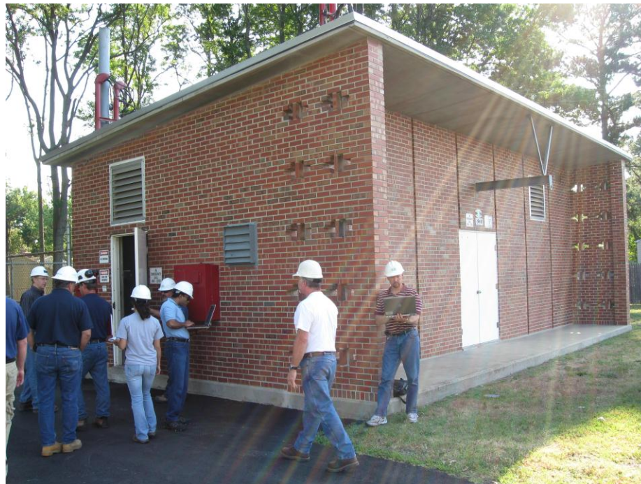
Figure 108-2. Dovercourt Rd Pump Station
