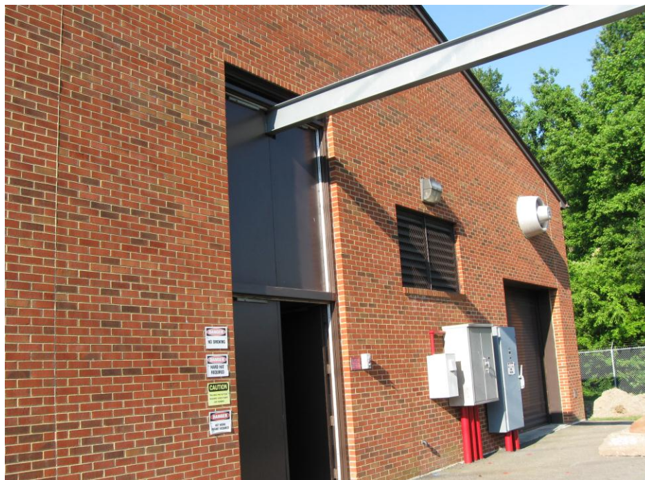
Figure 152-2. Terminal Blvd PRS
