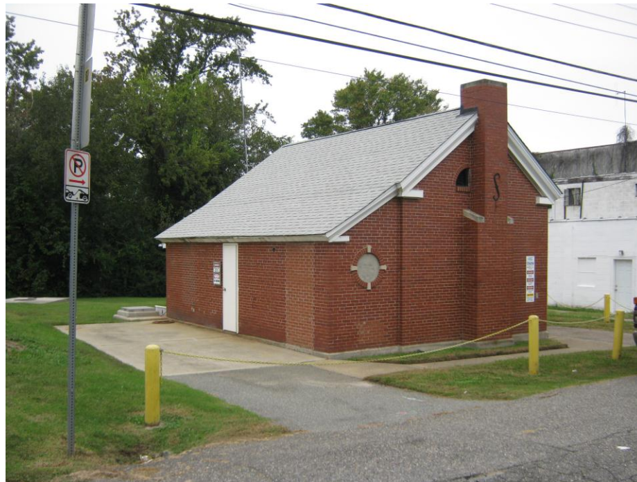
Figure 207-2. Center Ave Pump Station
