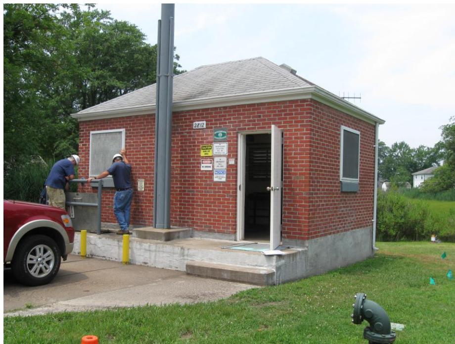
Figure 110-2. Ferebee Ave Pump Station
