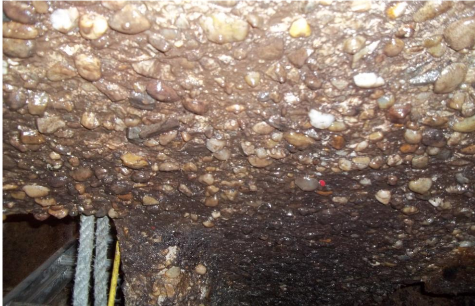
Figure 117-3. North Shore Rd Wet Well Ceiling
