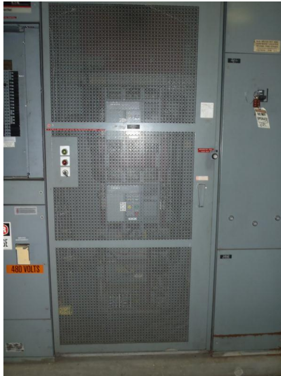
Figure 143-5. Transfer Switch
