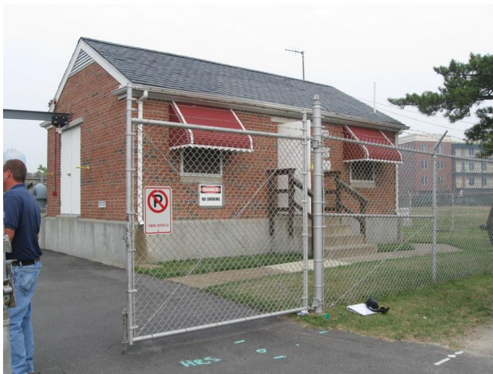
Figure 101-2. Arctic Avenue Pump Station
