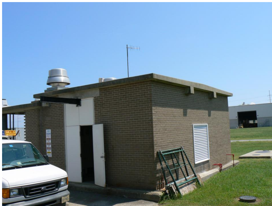
Figure 209-2. Copeland Park Pump Station
