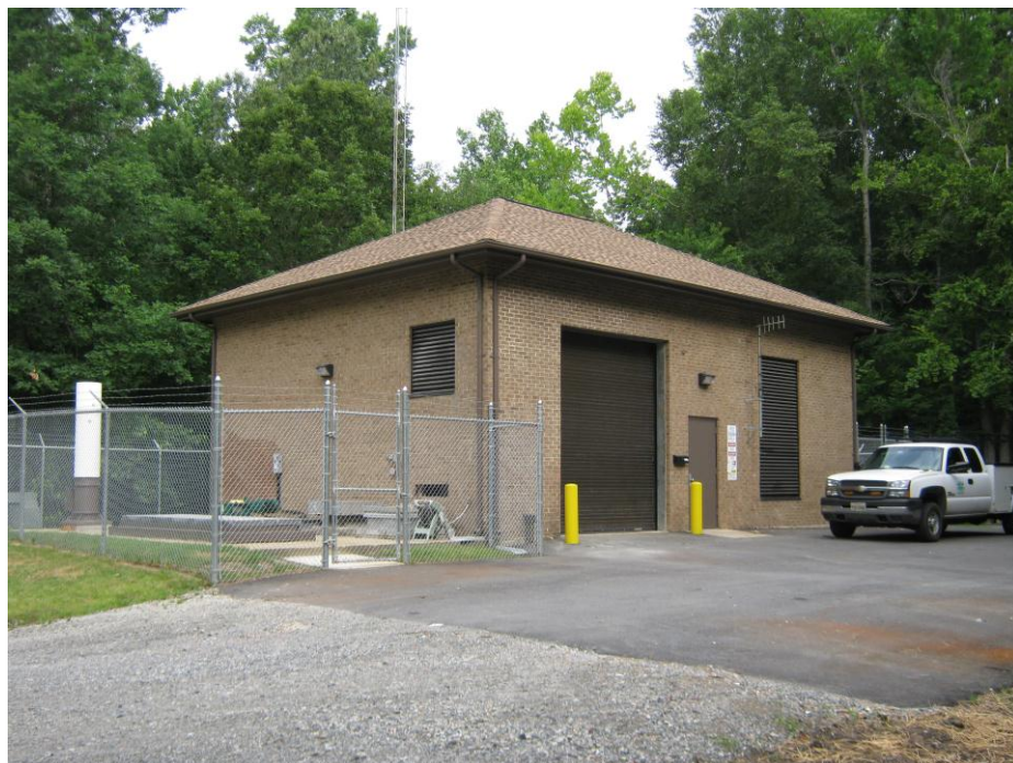
Figure 231-2. Fords Colony Pump Station
