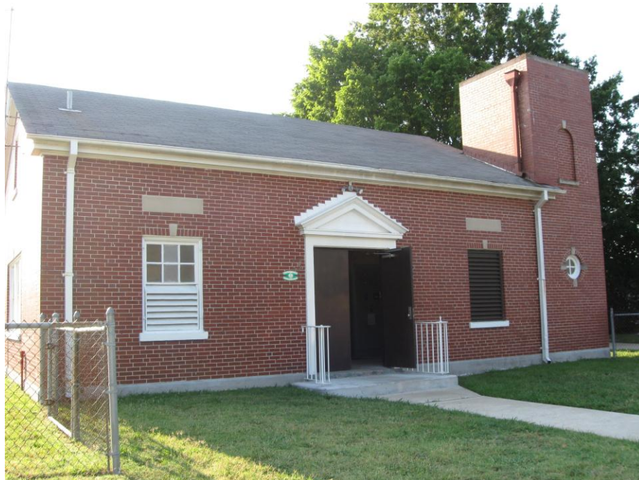
Figure 146-2. Camden Ave PS
