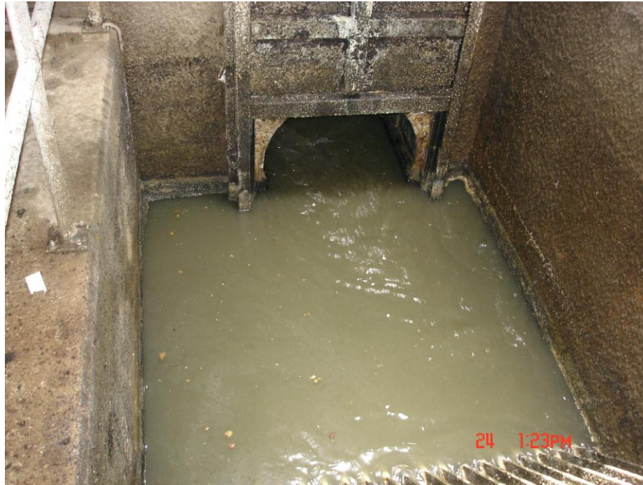
Figure 227-3. Ft. Eustis Influent Channel.
