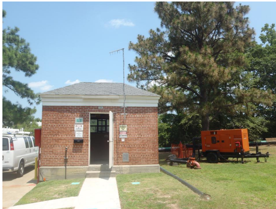
Figure 106-2. City Park Pump Station
