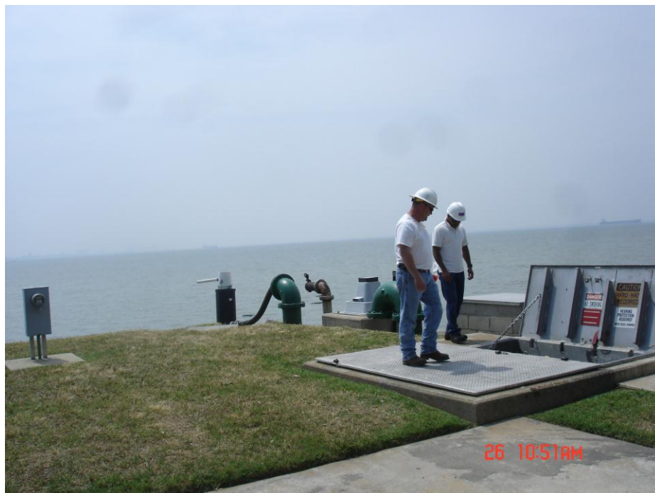
Figure 208-2. Claremont Ave Pump Station
