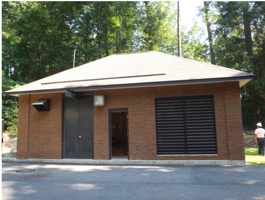
Figure 229-2. Colonial Williamsburg Pump Station
